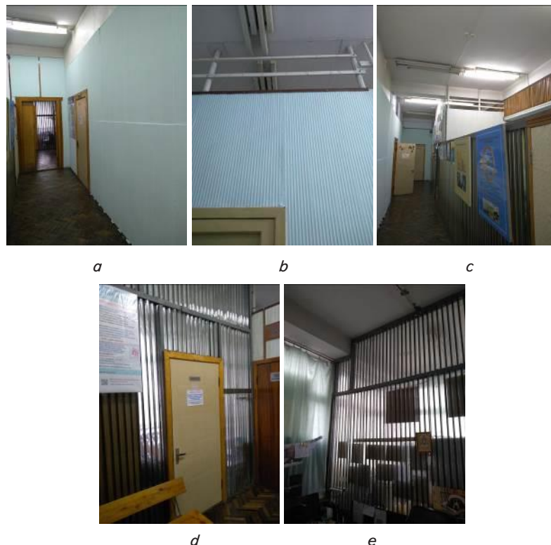
Fig. 2. Photographs of the rooms in the office of open space type with partitions: 100 % separation (ceramic panels and expanded polystyrene) (a); 75 % separation (ceramic panels) (b); 50 % separation (glass pipes with rubber gaskets) (c); 100 % separation (glass pipes with rubber gaskets) (d, e)
